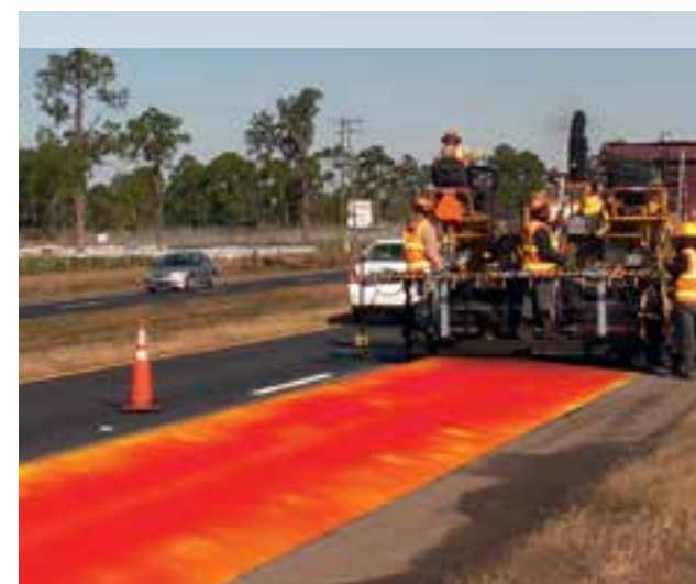
REAL-TIME INFRARED PAVER LEVELING
