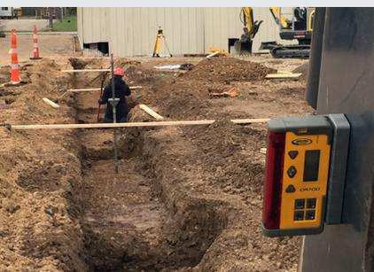
The Spectra Precision® CR700 Combination Laser Receiver is a machine mounted display receiver used on small grading and excavating equipment as well as a traditional laser receiver mounted to a grade rods. It is also ideally suited to work in vertical application for alignment control.
