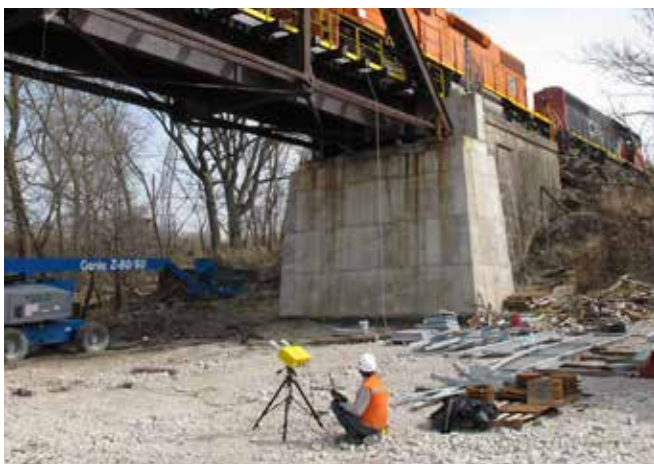
IBIS-FS monitoring an iron bridge
